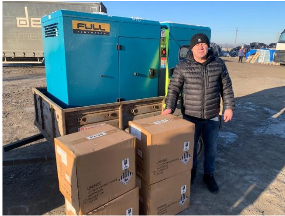
Kherson region, Petropavlivka village - Charging stations & generator 25kW
